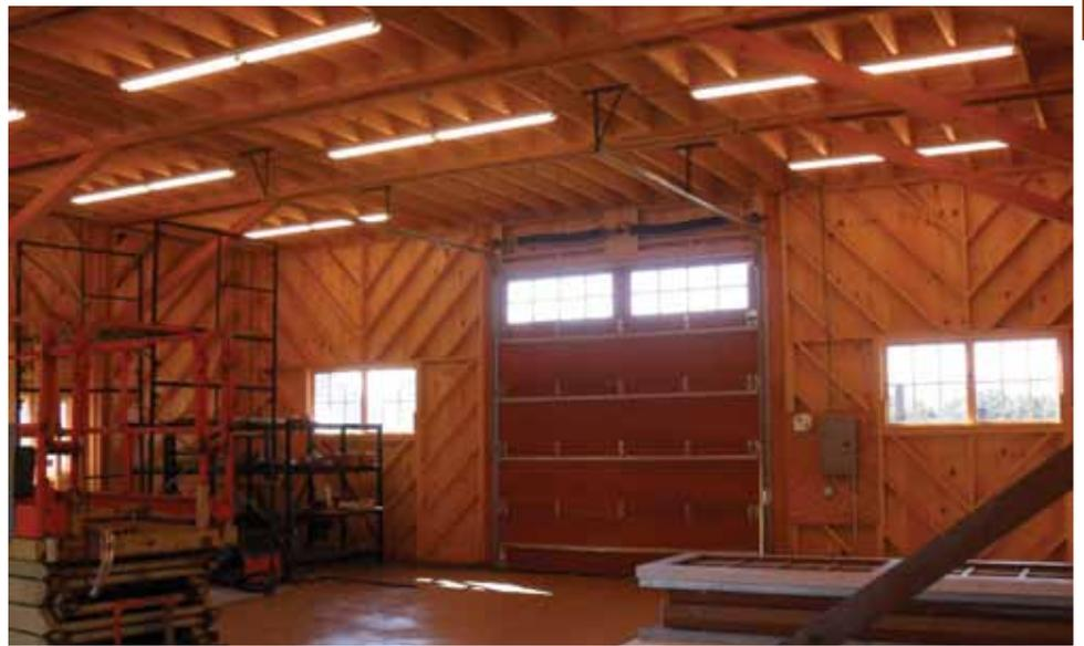
*The free spans above and below allow for complete versatility in the use of space without any interior columns or bearing walls.*
